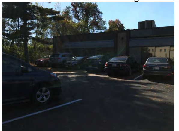
East Elevation and Parking
