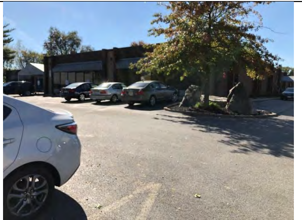
East Elevation and Parking
