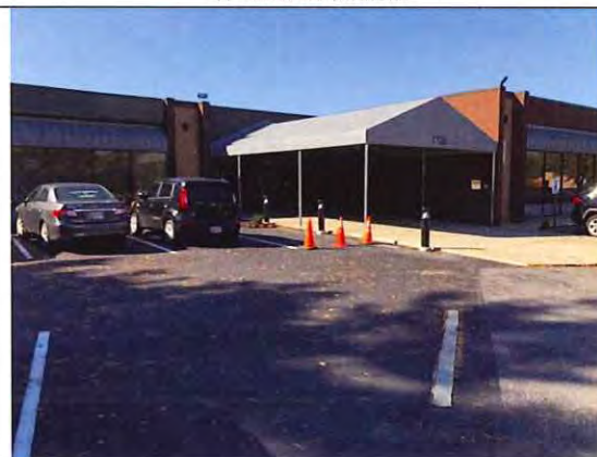
Current Front Entrance
