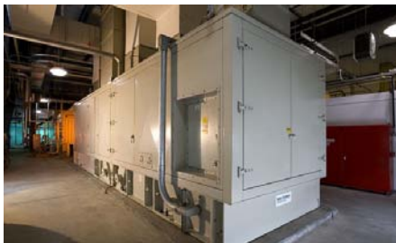
Combined Heat & Power (CHP) Systems
